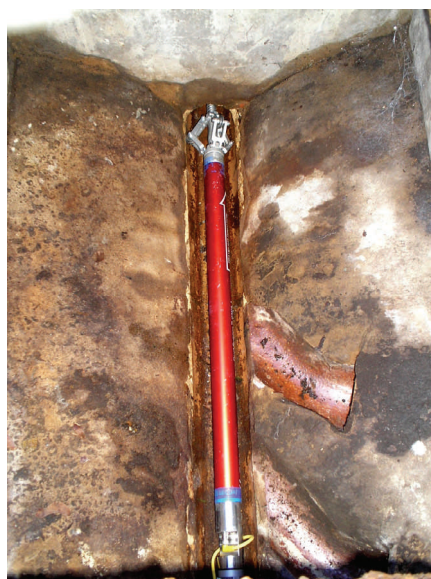
Left: Launching a PipeTrack unit from an existing manhole.
